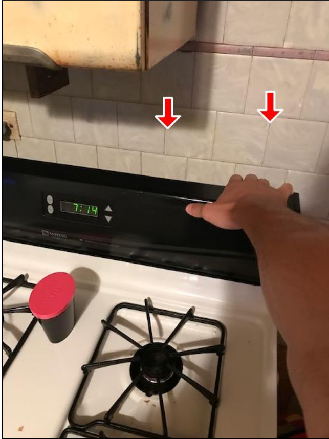
5.1 Item 1(Picture) Stove/Range is missing anti tip bracket. Safety hazard.
