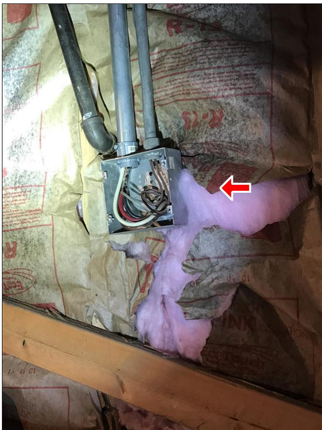
2.3 Item 2(Picture) Open junction box. Have a licensed contractor install cover. Shock hazard.
