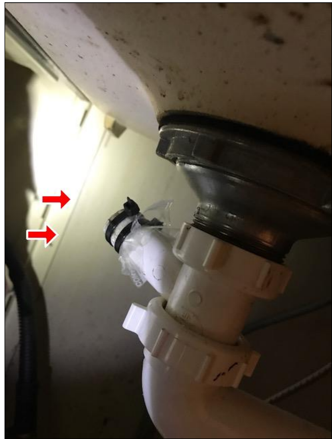
5.0 Item 2(Picture) Dishwasher line disconnected. Have qualified plumber repair or replace as needed.
