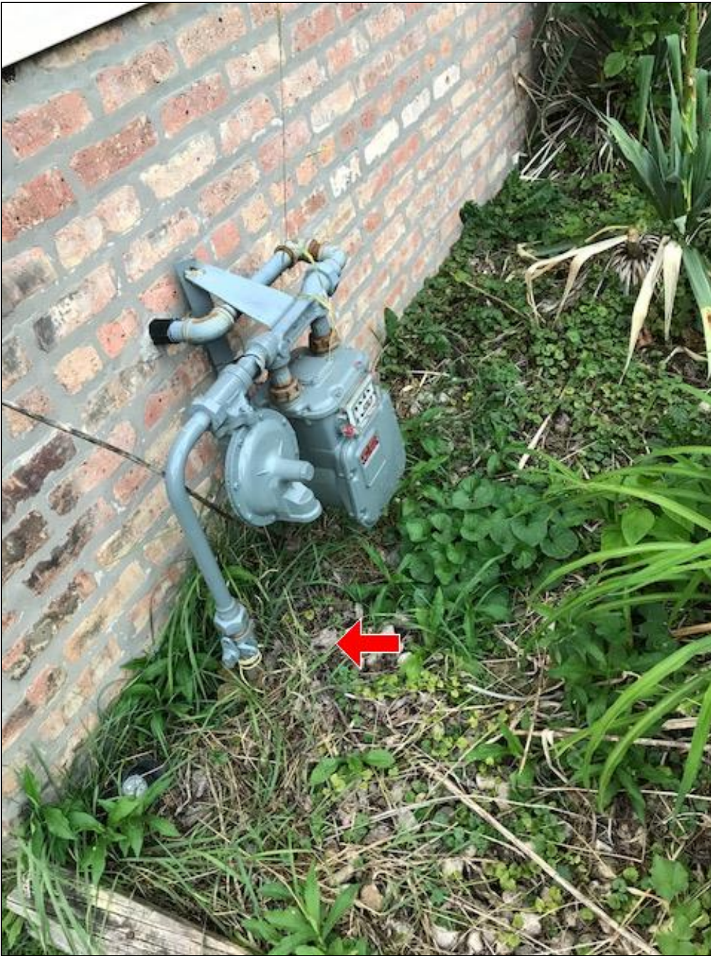
4.5 Item 1(Picture) For your information only: Main fuel shut off for house.
