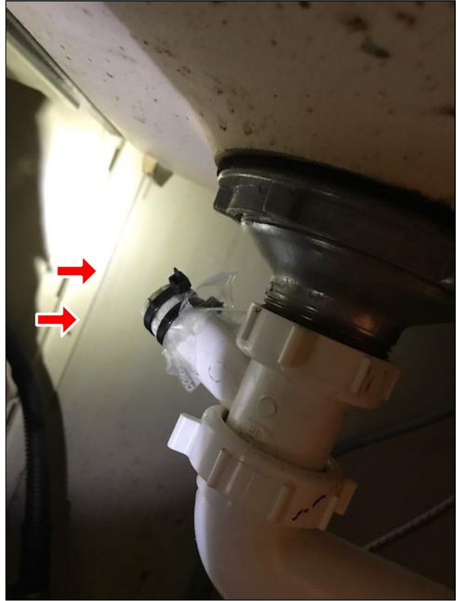
5.0 Item 2(Picture) Dishwasher line disconnected. Have qualified plumber repair or replace as needed.
